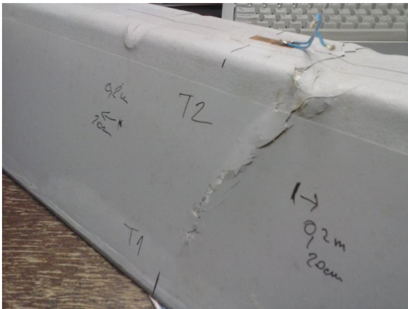
Figure 7. Failure of the carrier at the point of the force input.
