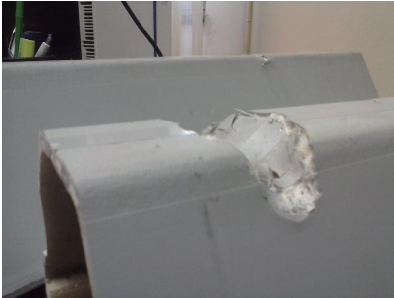
Figure 6. Failure of the carrier at the support.
