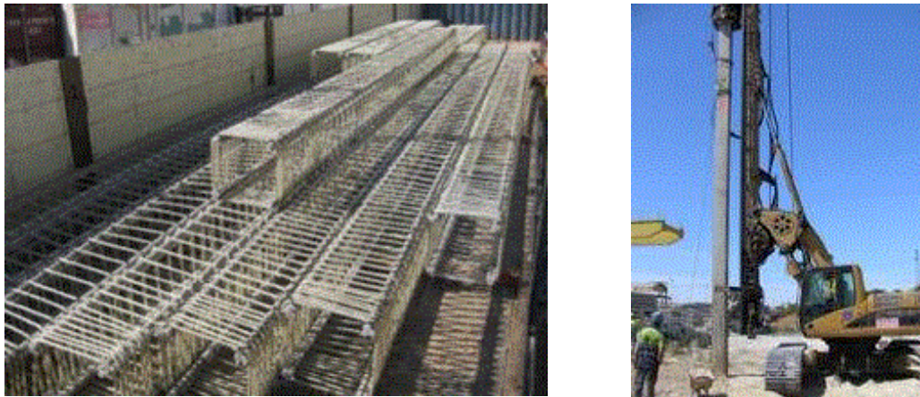
Figure 3. a) GFRP piles reinforcement cages; b) Pile P5 during its driving.
