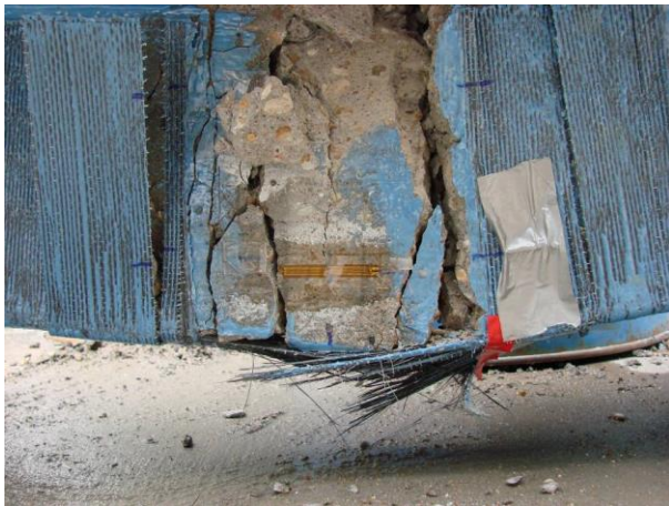
Figure 6 Beam T3 at failure
