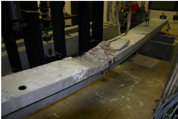
Figure 2 Beam T1 at failure
