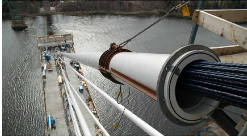
Figure 1. CFRP Cable strands into a cable stay bridge in Maine (USA) [4].
