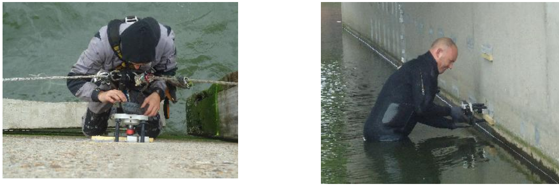
Figure 6 : Pull-off test: (a) on the quay wall, and (b) at the bridge abutment
