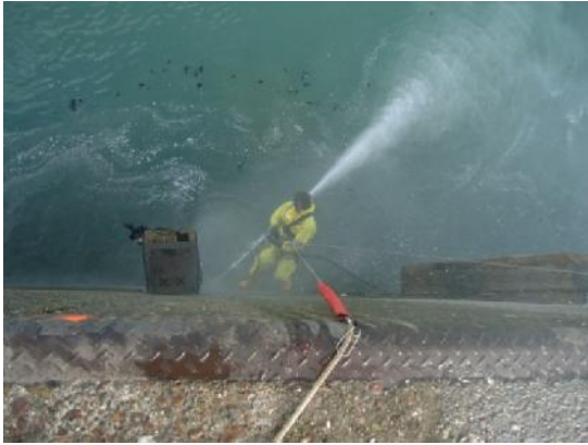
Figure 3: Surface preparation using pressured washed
