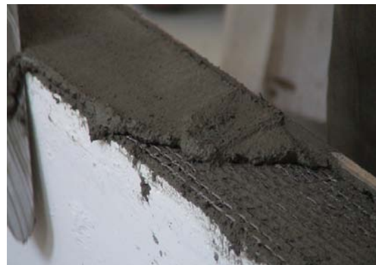
b) Application of second layer of mortar
