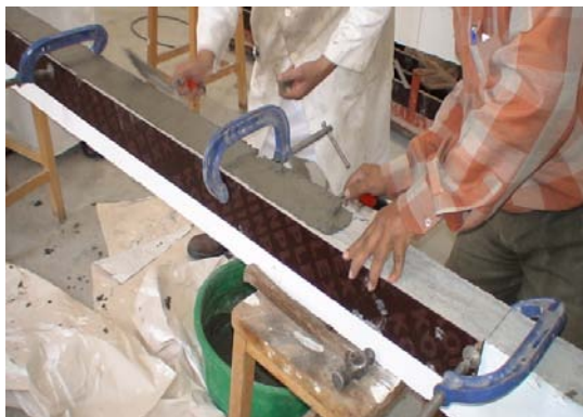
a) Application of first layer of mortar
