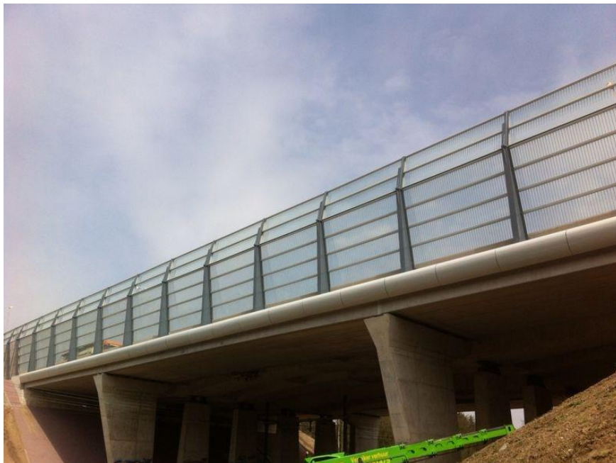
Figure 12. Edge elements installed on the bridge
