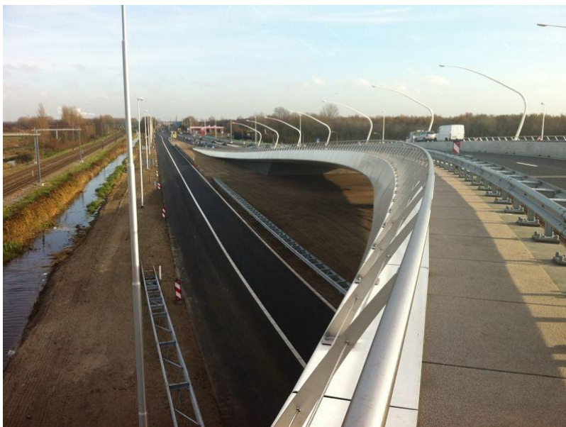
Figure 18. Edge profiles installed on the fly-over
